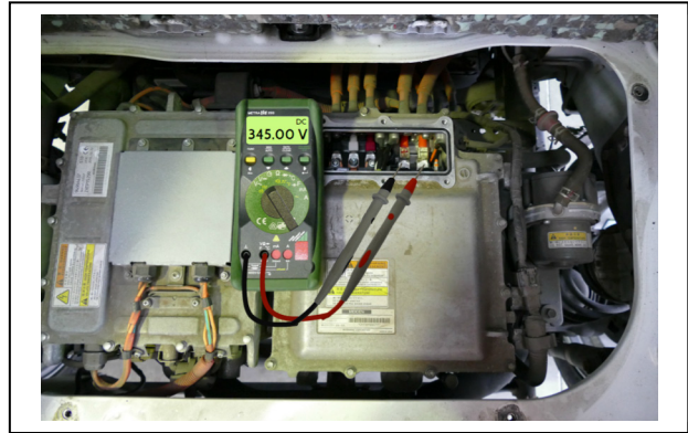
Figure 10: Interactive measurement at the inverter of an EV
