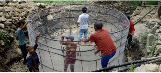
Figure 7. Constructing a new rainwater tank in Sandikohla, 2013
