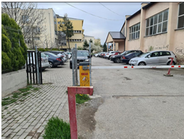
Fig. 3. Parking of vehicles with entry-exit barriers
