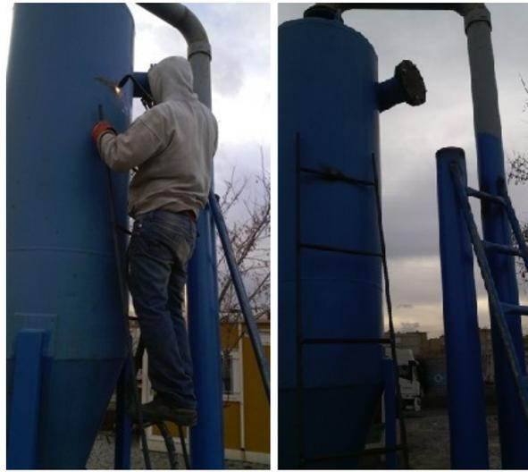
**Fig. 3.** Stages of cutting inlet gate to hydrocyclone
