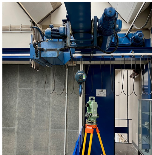
Fig. 1. Real experiment with a theodolite—measuring the deflection of a crane bridge
