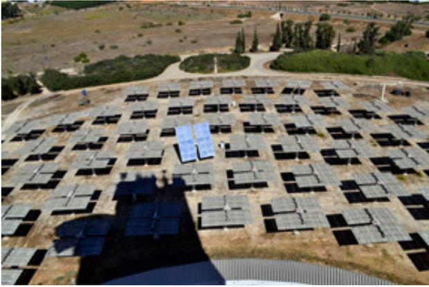
Figure 3. Heliostats field
