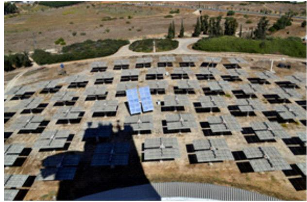
Figure 2. Heliostats field
