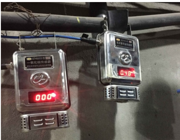
Figure 4. Site installation of methane sensors
