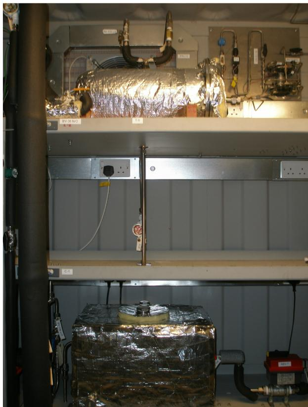
Figure 3. Photograph of the Flue Gas Conditioning and Distribution Infrastructure showing the knockout drum at on the top shelf, the water inventory tank on the lower shelf and the spray column on the left
