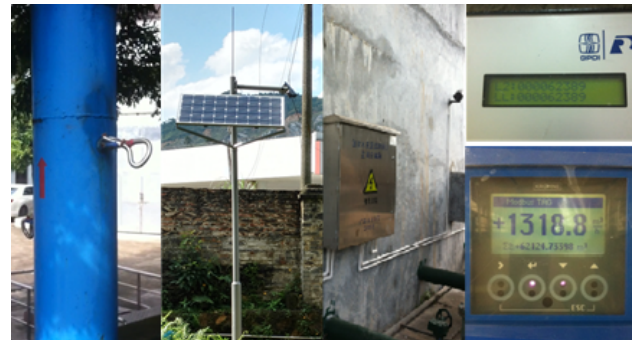
Figure 11. Instrument installation in the field
